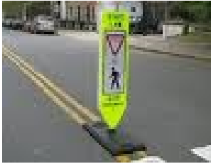
In-road YTP sign
