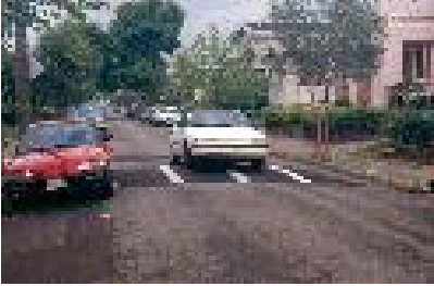
Asphalt speed hump
